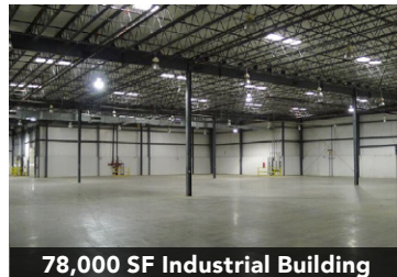
78,000 SF Industrial Building
