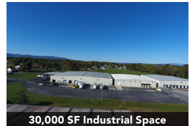
30,000 SF Industrial Space
