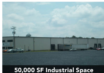
50,000 SF Industrial Space
